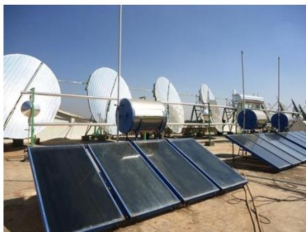
*Photo: A combination of low temperature and medium temperature solar thermal systems at an industry in India*
