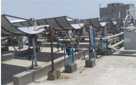
*Photo: Parabolic trough process heat at Amul Dairy, Gandhinagar*
