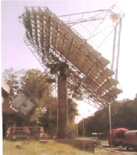
The Aurangabad plant of Bajaj Auto Limited (BAL), has commissioned the Arun160™ dish concentrated solar thermal water heating system integrated into its existing Liquefied Petroleum Gas (LPG) for meeting its process heat requirements.
