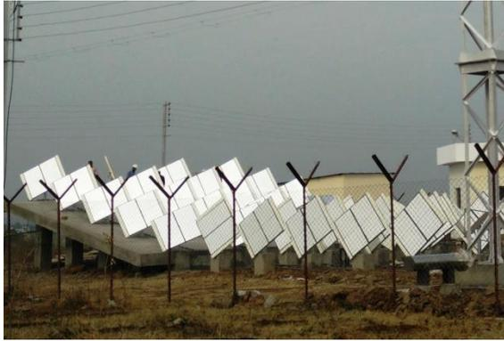
*Photo: 30 kW-thermal CLCSP system, courtesy, RGTU, Bhopal*
