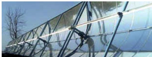
Each single module of a SolPac P60 (6.41m<sup>2</sup>) needs a shade free area of 10m<sup>2</sup> and weighs 250kg. It has an output capacity of 1.4 to 1.8kW<sub>th</sub>. Thus, the total shadow free area requirement for 40 modules is around 400m<sup>2</sup> and weighs 10 tonnes.
